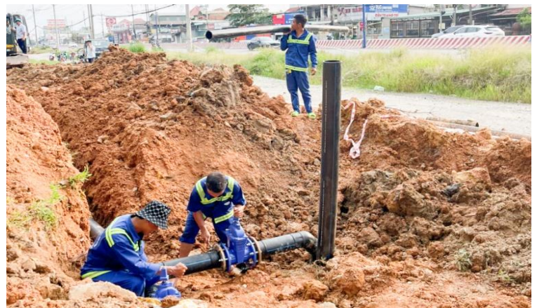
Relocating the water supply system on Binh Duong Boulevard
