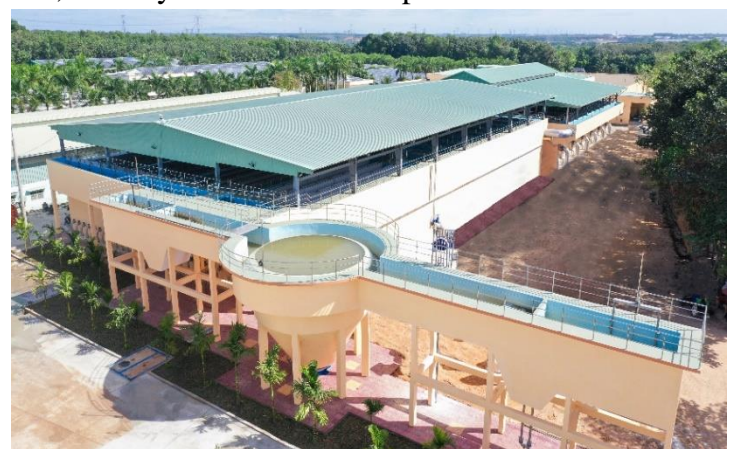
Tan Hiep Water Plant, phase 3, has an additional capacity of 100,000m 3 /day and night to meet the development needs of the province
