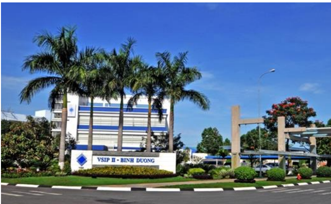
Attracting FDI and large investment projects in Binh Duong will increase the demand for clean water
